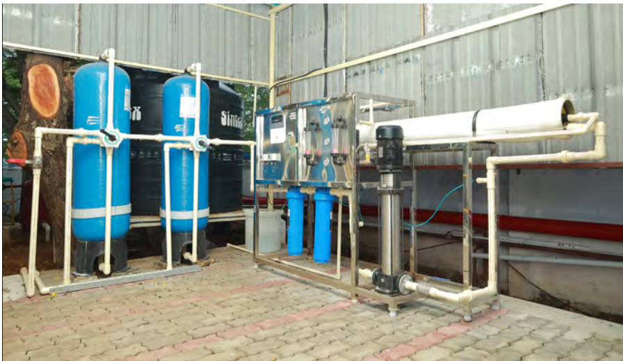
RO system for ETP treated water -Savings – 10KLD
